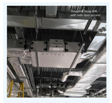
Adapting to New Technology. By taking a decentralized approach to ventilation, each energy recovery unit (ERV) delivers fresh, filtered outside air directly to the classroom, while stale air is exhausted. Decentralized ventilation eliminates the need for vertical duct chases, rooftop units and bulky equipment. Low-profile ERVs can be floor, wall or ceiling mounted to fit into drop ceilings and mechanical rooms with limited space.
