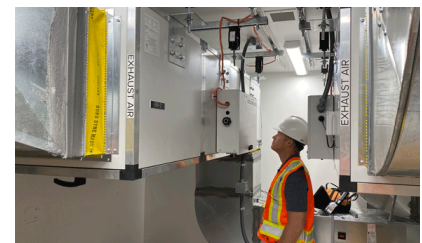
University Residence Retrofit | Kelowna, BC Nova C24 & C30 | 8100 cfm
