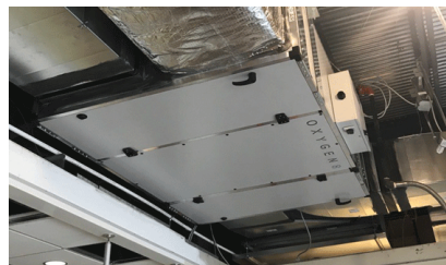
Office Retrofit | Boston, MA | Nova C24 | 1500 cfm
