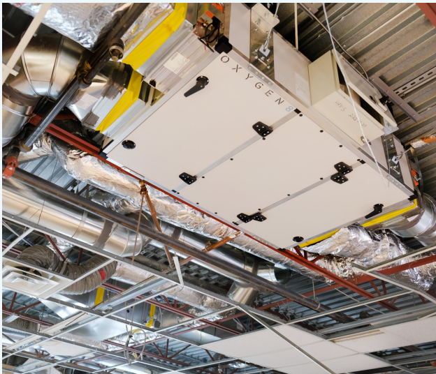
Oxygen8 Nova DOAS ventilating the activities and crafts room at a British Columbia senior care facility.
