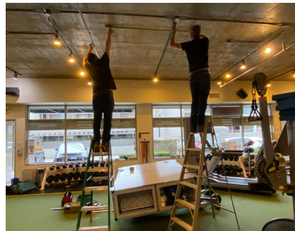
Ceiling Mounting the Ventum ERV
